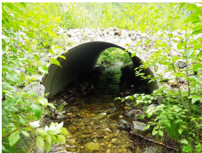
Two examples: Left - what we don't want in our waterways, a perched culvert and above - what we do want - stream simulation
