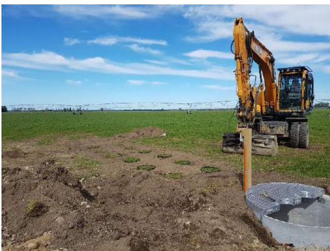
Lysimeter installation.
